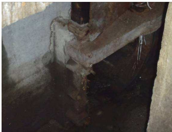
Vanne exutoire principal
